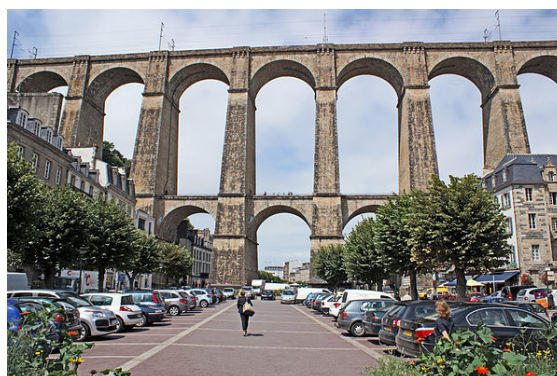
The Morlaix railway viaduct is one of the highest in France.
